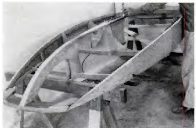
GLUE IS APPLIED and keel is sprung into position. Use clamps to hold forward deck-beam blocking
